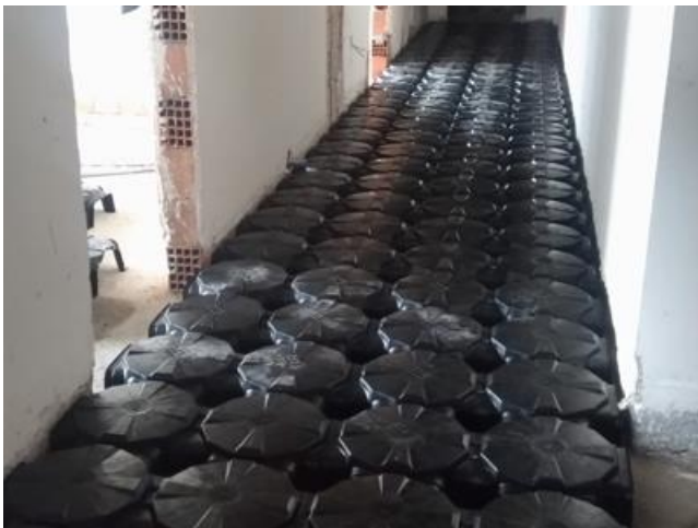
ELEVATOR, STAIRCASE, HALLWAY FILL
