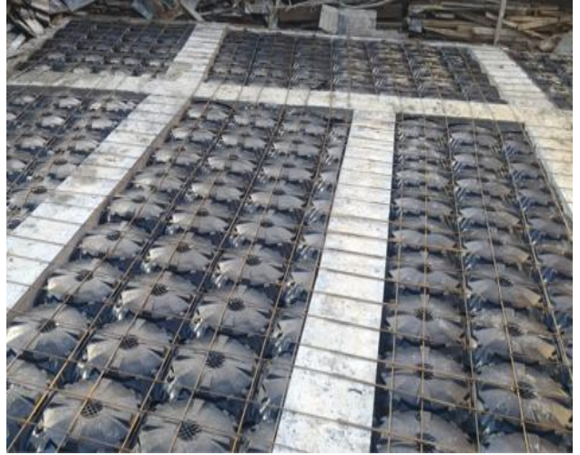
INVERTED BEAM FILL
