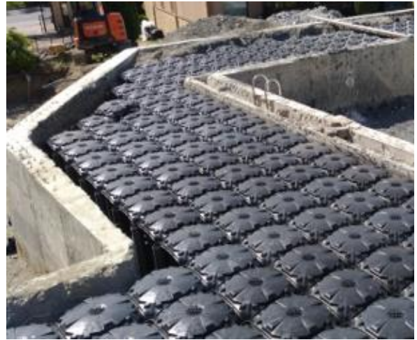
POOL DECK SLAB FILL
