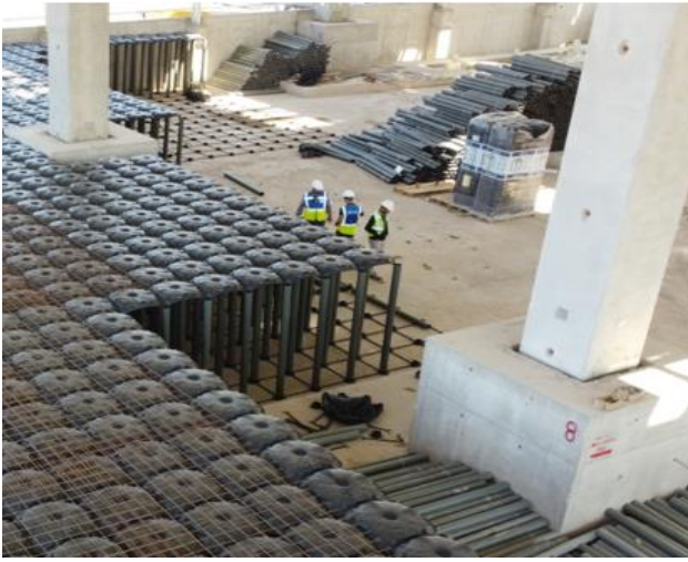
FILL BETWEEN FOUNDATION FOOTINGS
