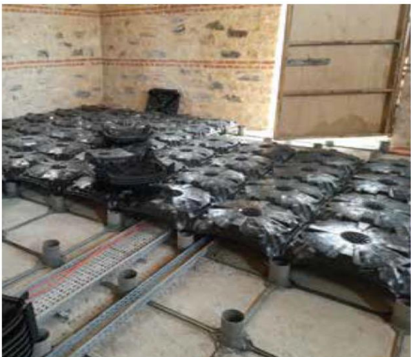
CONCRETE RAISED FLOOR AND INFRASTRUCTURE CONSTRUCTION
